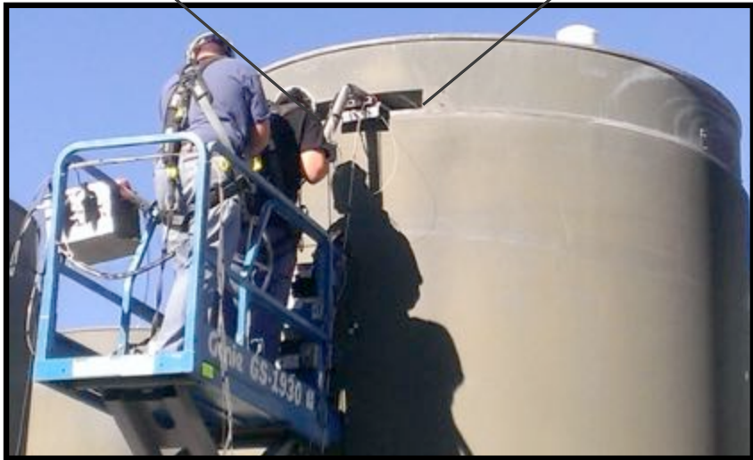
Example robotic inspection of DC ISFSI system
