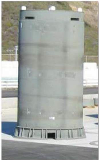
Figure 8: HI-STORM 100SA System
