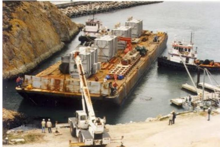
Figure 11 - Use of Barges to Bring in Materials - 1994
