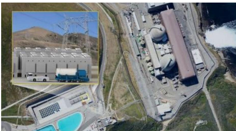
Figure 20 - NUHOMS® Used Fuel Storage System shown in the existing ISFSI
