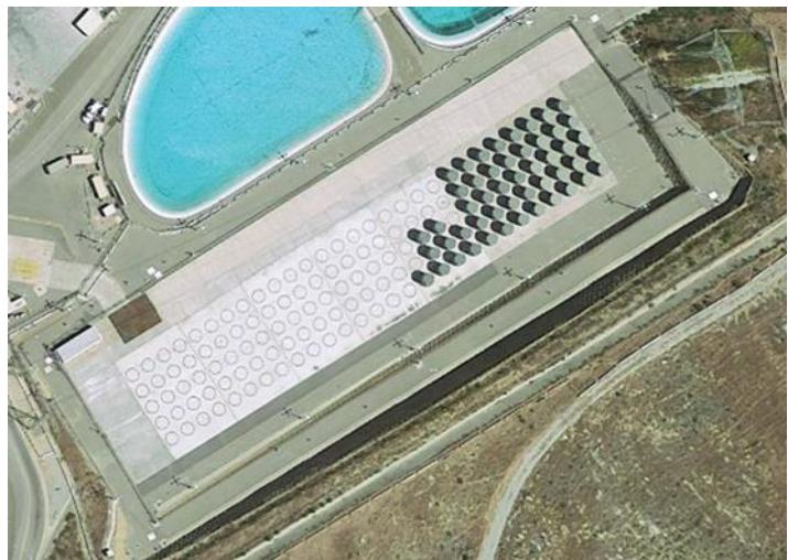
Figure 9: DCP ISFSI Pad in 2017 with 49 Loaded Casks
