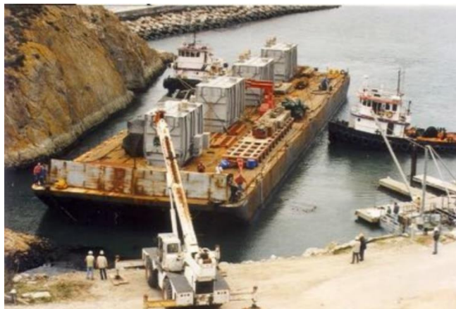
Figure 11 - Use of Barges to Bring in Materials - 1994
