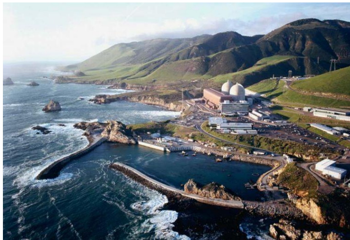
Figure 10 - East and West Breakwater and Harbor Area
